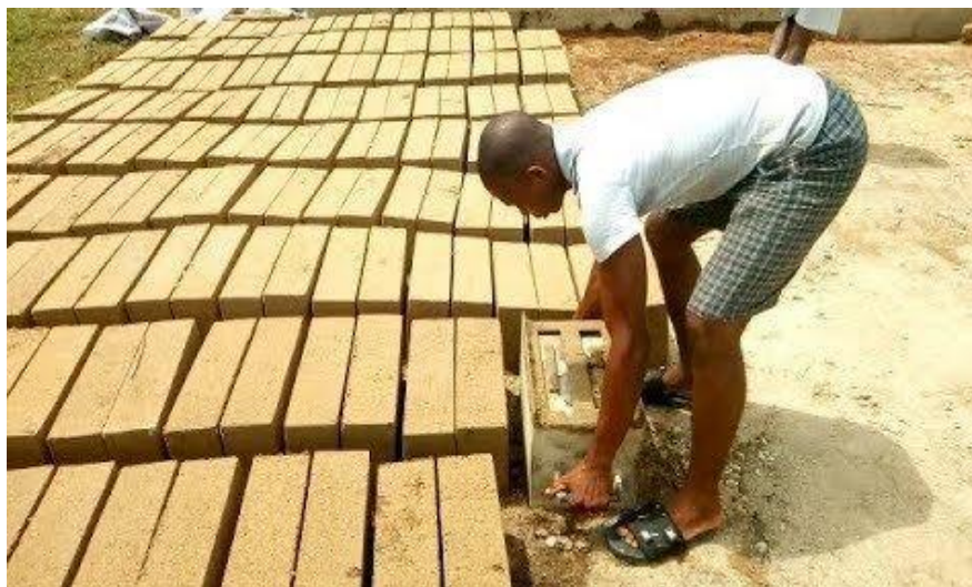
Figure 2: Hand moulding of blocks
