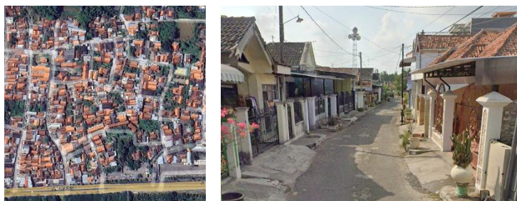
Figure 10. Aerial view of the city center district; and Figure 11. The city center district
